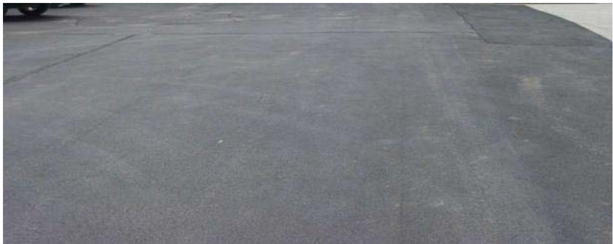
Figure 11. Pavement constructed in 1972 with GSB-78 applied every four years.
