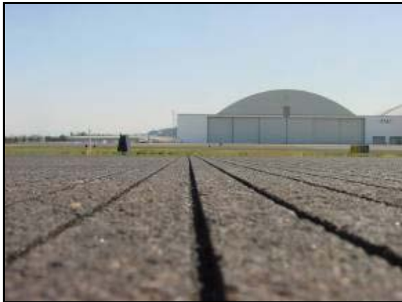
Figure 5. Groove remained sharp and clean.
