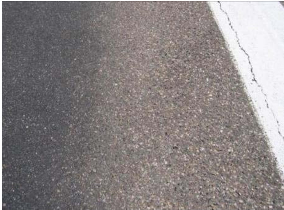
Figure 36. Pavement generated FOD on non-treated pavement.
