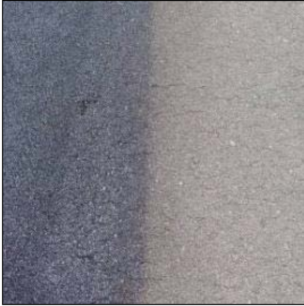
Figure 40. GSB-88 seals ‘checking’ cracks.
