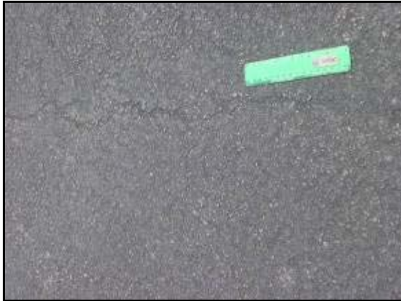
Figure 12. GSB-78 has kept cracks sealed.
