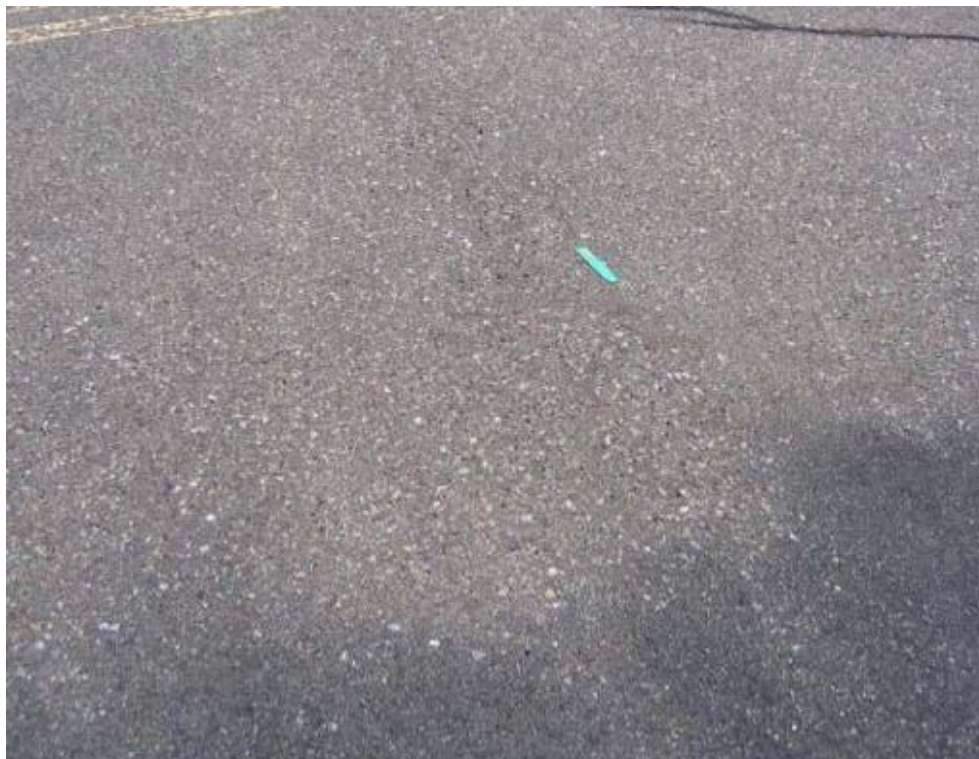
Figure 37. Pavement generated FOD on non-treated pavement.
