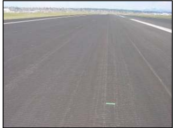
Figure 4. PDX grooved runway with GSB.
