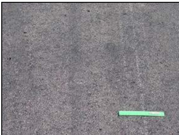
Figure 7. Holes from dissolving aggregate.
