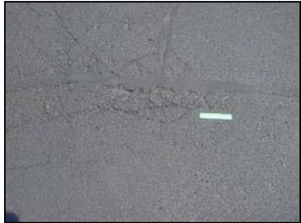
Figure 17. GSB seals and protects from water intrusion.
