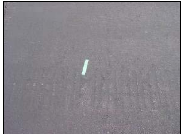
Figure 35. Pavement scars treated with GSB.
