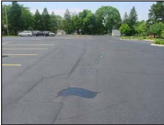
Figure 16. GSB will not stop structural distress.
