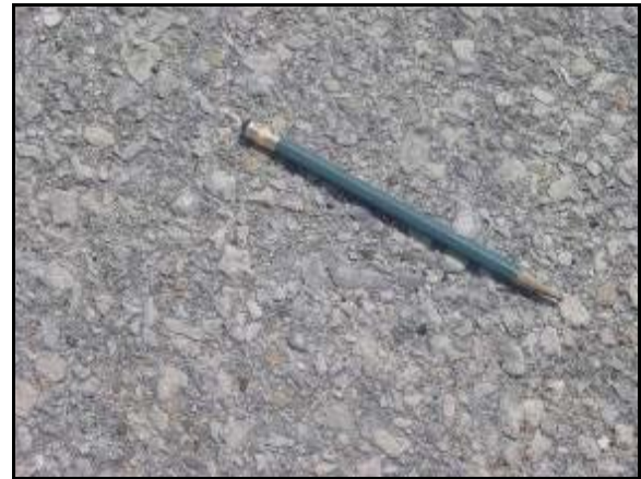
Figure 15. No treatment results in raveling.
