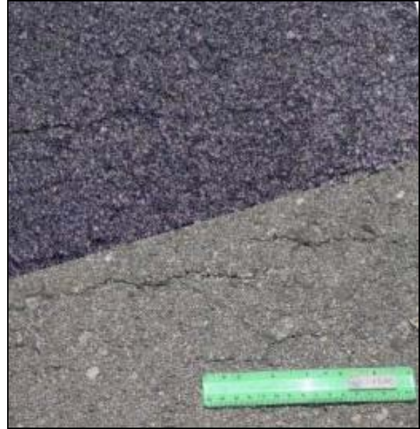
Figure 41. ‘Checking’ and hairline cracks.
