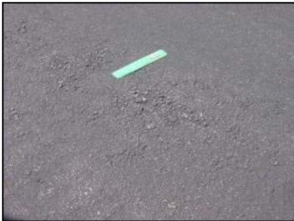
Figure 34. Segregation treated with GSB.
