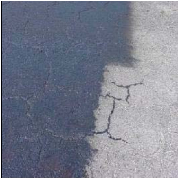
Figure 38. Cracks filling at edge of application.
