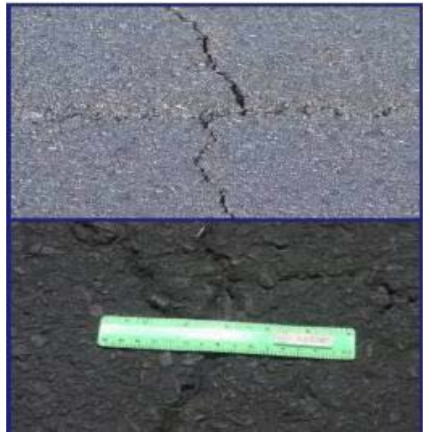
Figure 39. Partial filling with one coat.
