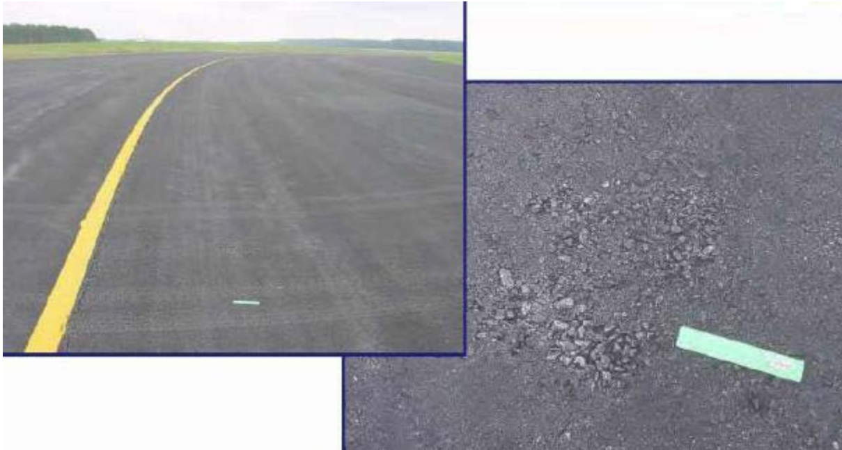
Figure 33. GSB-88 applied to segregated area, resulting in control of pre-raveling.
