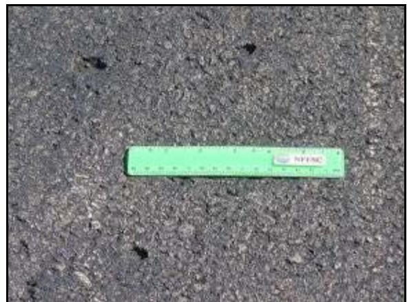
Figure 8. Holes sealed from water intrusion.
