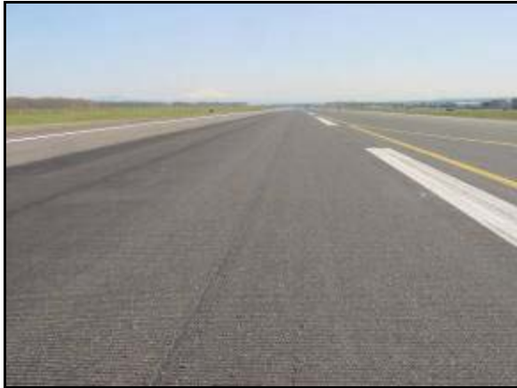
Figure 3. PDX grooved runway with GSB.
